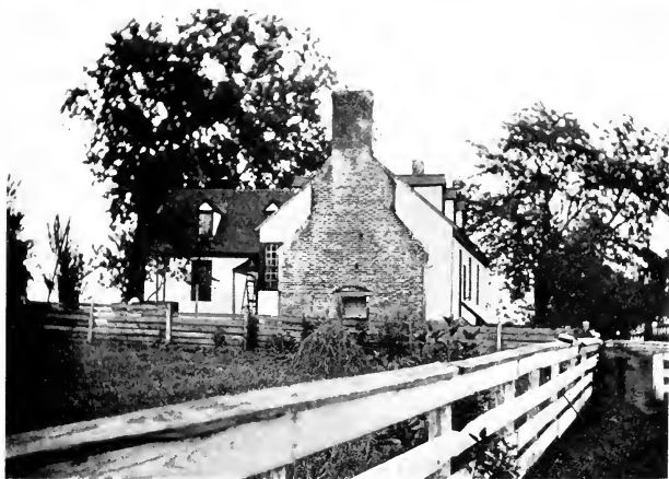
THE ROBERTSON HOUSE, CHESTERFIELD COUNTY. BUILT ABOUT 1750 Frame dwelling with chimney twenty-five feet wide
